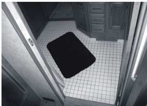
A simple rubber-backed rug covers the drain when shower is not in use. View from living area doorway.
