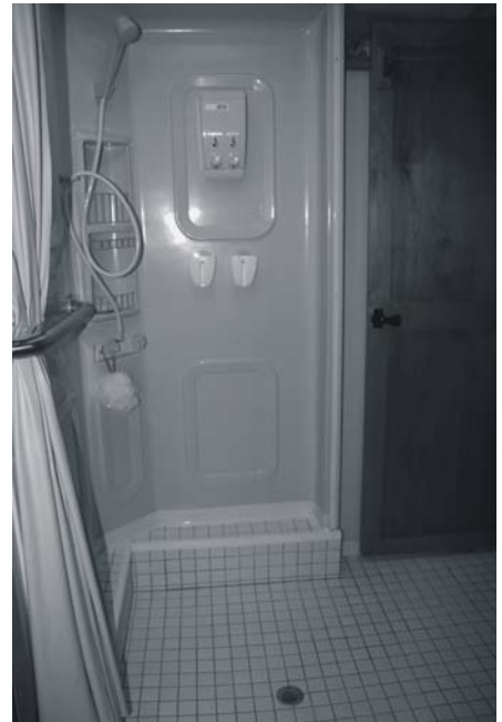
View of new shower as seen from WC. Shower curtain on left is tucked behind the safety bar when shower is not in use.
